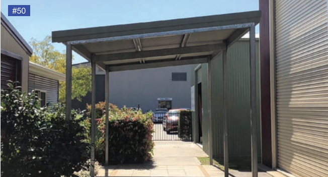
Mist Green roof, gutters.
