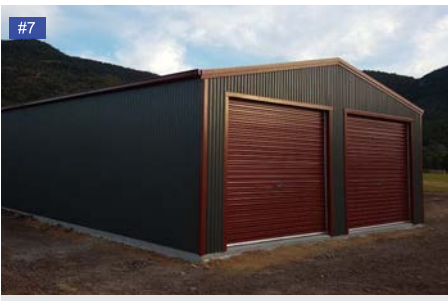
Monolith walls, Heritage Red gutters, roller doors.
