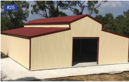
Smooth Cream walls, Heritage Red gutters, roller door.
