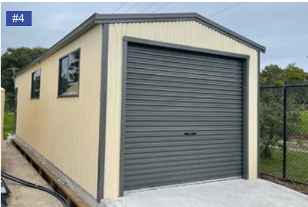
Smooth Cream wall, Slate Grey gutters roller door.
