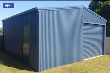
Mountain Blue walls, gutters, roller doors.
