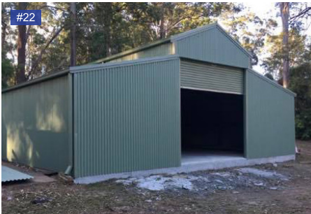
Mist Green walls, gutters, roller door.
