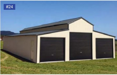
Smooth Cream walls, Slate Grey gutters, roller doors.
