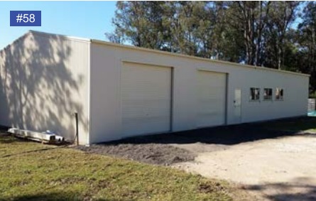
Smooth Cream walls, gutters, roller doors
