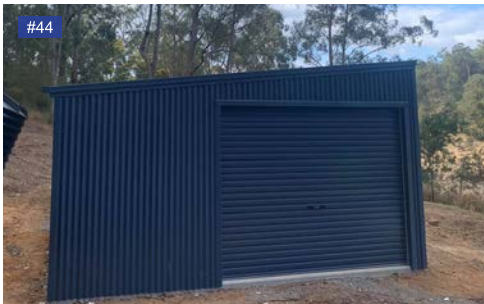
Mountain Blue walls, gutters, roller doors.
