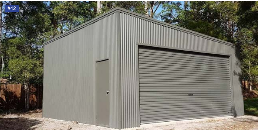
Slate Grey walls, gutters, roller door.
