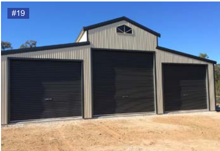
Smooth Cream walls, Monolith gutters, roller doors.
