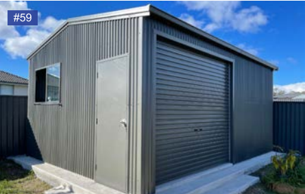
Slate Grey walls, gutters, roller doors.
