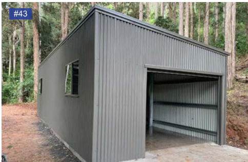
Slate Grey walls, gutters, roller door.
