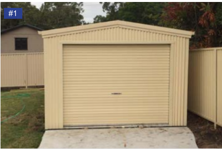
Smooth Cream walls, gutters, roller door.
