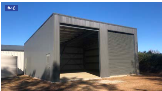
Slate Grey walls, gutters, roller door.
