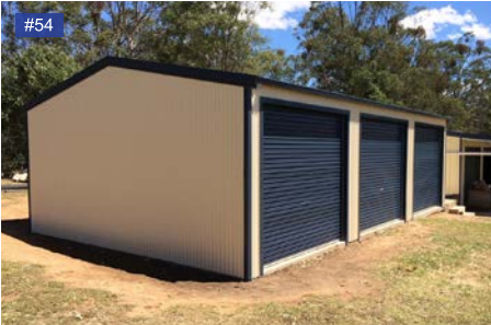
Smooth Cream walls, Mountain Blue gutters, roller doors.
