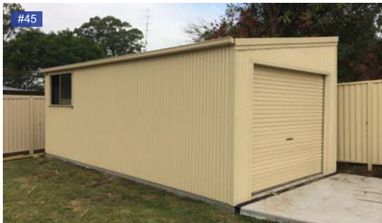
Smooth Cream walls, gutters roller door.
