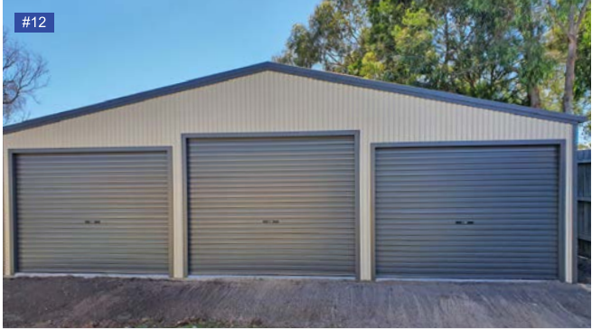
Smooth Cream walls, Mountain Blue gutters, roller doors.
