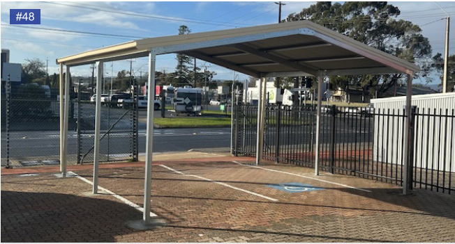
Smooth Cream roof, gutters.
