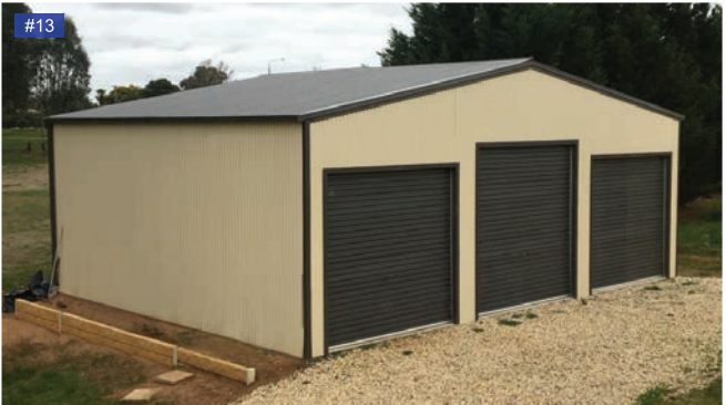
Smooth Cream walls, Slate Grey gutters, roller doors.
