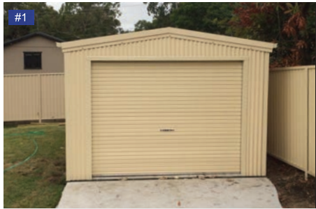
Smooth Cream walls, gutters, roller door.
