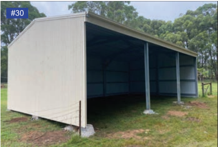
Smooth Cream walls, gutters.
