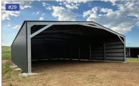
Monolith walls, gutters.
