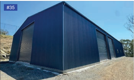
Mountain Blue walls, gutters, roller doors.
