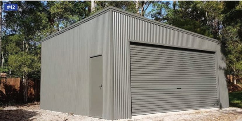
#42 Slate Grey walls, gutters, roller door.
