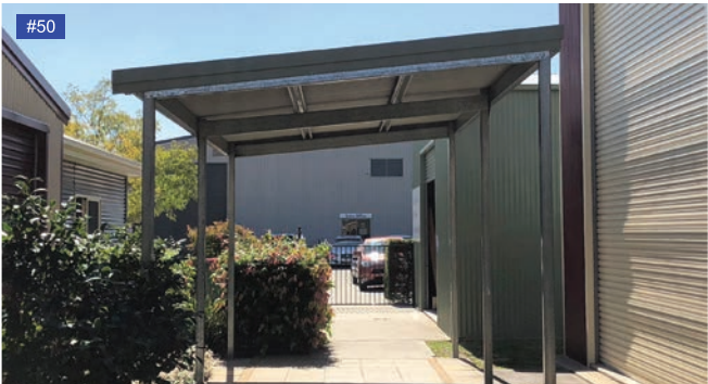
Mist Green roof, gutters.
