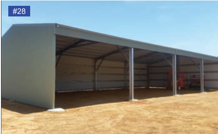
Mist Green walls, gutters.
