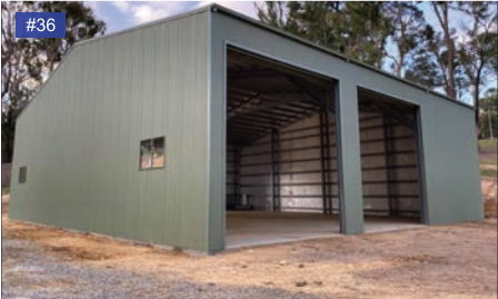
Mist Green walls, gutters, roller doors.
