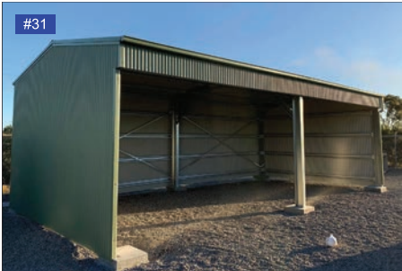
Mist Green walls, gutters.
