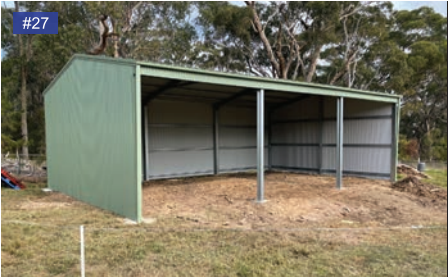
Mist Green walls, gutters.
