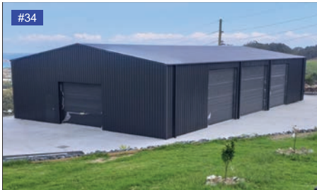
Mountain Blue walls, gutters, roller doors.
