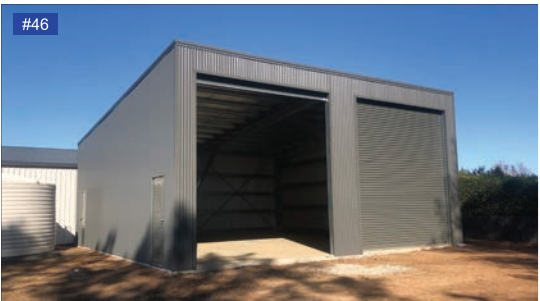
#46 Slate Grey walls, gutters, roller door.
