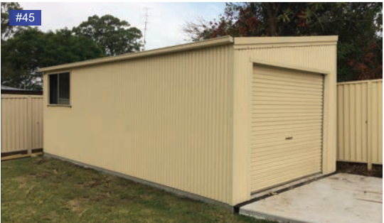
#45 Smooth Cream walls, gutters roller door.
