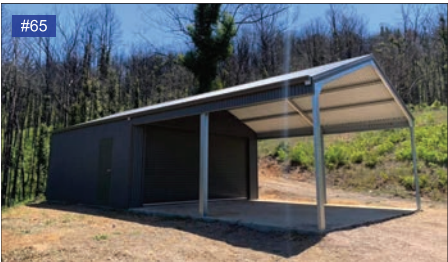
Monolith walls, gutters, roller doors.
