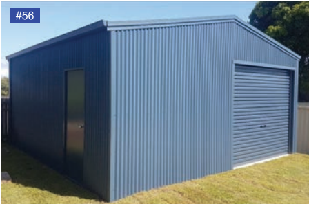
Mountain Blue walls, gutters, roller doors.
