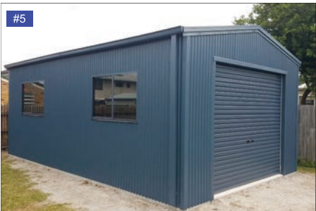
Mountain Blue walls, gutters, roller door.
