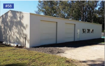
Smooth Cream walls, gutters, roller doors
