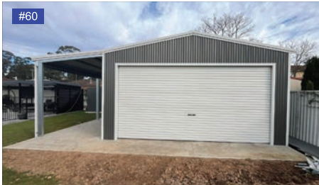
Slate Grey walls, Off White gutters, roller doors.
