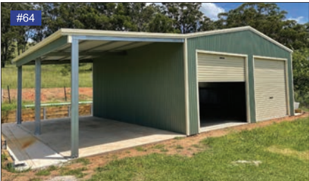
Mist Green walls, Smooth Cream gutters, roller doors.
