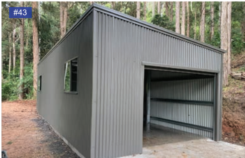
#43 Slate Grey walls, gutters, roller door.
