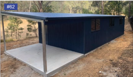
Mountain Blue walls, gutters, roller doors.
