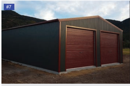
Monolith walls, Heritage Red gutters, roller doors.
