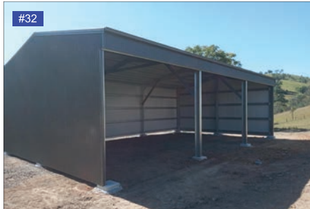
Slate Grey walls, gutters.
