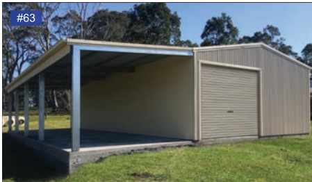
Smooth Cream walls, gutters, roller doors.
